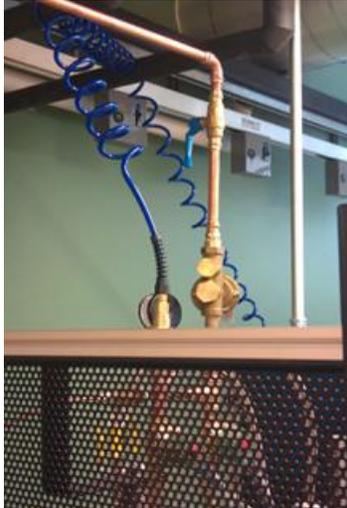
12. The water valve on the back of the machine (labeled 5) should be closed.
